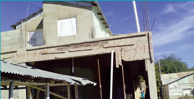
Above Left and Right: A new area was created in the second story as the concrete slab that serves as the second story floor was poured. The new area in the first story is space for the water purification system.
