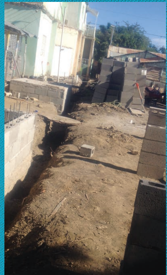
Below Right: Cement cinder blocks sit next to the new construction.
